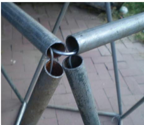
As a further vision, consider again the hexagonal enclosure. If you wired in six tubes of adequate lengths to a point in the center you could create a roof frame for the encircling triangles. Note that these six tubes would need to be longer than the tubes of the surrounding hexagon, or the surface would remain flat. So a minimum of two tube lengths will be needed for this
