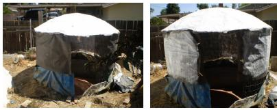
After the final coat on the top, I wired it to the fence material and wrapped the side with the weed block matting. I found clothes pins helpful in securing this matting to the sides. I also applied small dollops of undiluted paint to the wire and matting from inside, to better secure
