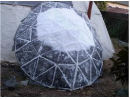
I left a little bit of this roofing material protruding from the edge of the frame, to shed runoff.
