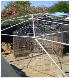
The top is a dome fabricated from pieces of #9 gauge steel wire welded together. This wire is commonly used to help stiffen the bottoms of chain link fences and is widely available at home improvements stores. The wall is 25' of 5'-high wire fencing.
