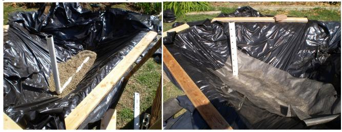
After back filling the bed, fifteen gallons of water were poured down the riser. A water depth of about a foot was measured by a wooden dipstick.
