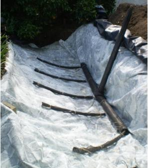
I've created an impervious liner for this garden, by painting a tough (15-year guarantee) weed block material to 6 mill black plastic, using a solar roof coating material (10 year guarantee under outdoor weather conditions).
