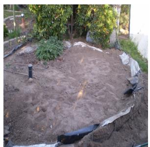
Additional membrane material was attached, and the enclosed area was back filled to the former grade. A pile of leaves was spaded into the newly back filled portion.
