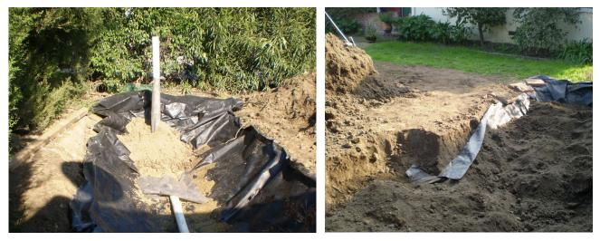
Rather than terminate the edge abruptly at 12" below the surface, I allowed a foot of it to extend horizontally, so it could overlap with any future trenches.
