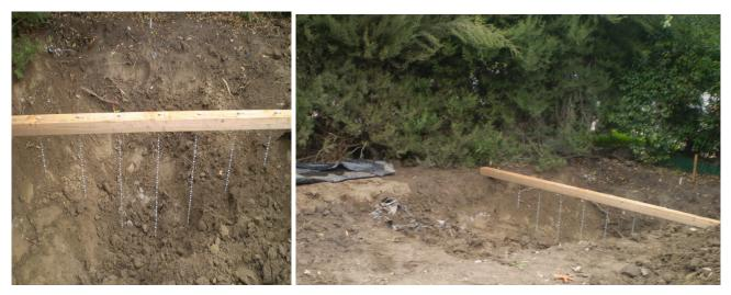
I chose to slope the bottom towards the riser by about ½" per foot (purely arbitrary, but I assumed the water would be intelligent enough to take the hint). I temporarily installed three 12 inch pavers at the ends and middle points to guide me in keeping this slope line straight.
