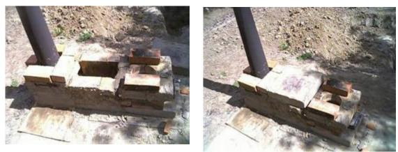
If you are installing a cooking surface, add some bricks or other obstacle for the flue gasses to jump over, so they will be forced to travel against the bottom of the plate.
