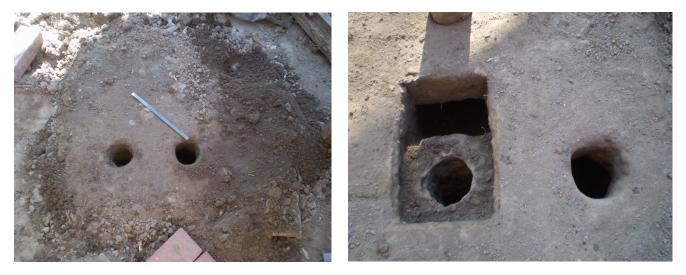
By digging downward at the other end I was able to make a channel to a third 3" hole, to which I connected the 3" flue pipe. In order to not dissolve everything by accidentally spilling something on it I solidified the structure by firing it. I did this by covering the rectangular hole with bricks to trap the heat, limited spare drafts by pouring on a little dirt, and built a fire.
