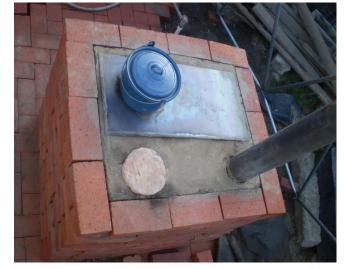
There is more to this stove than just a pretty face. I have intentionally built in an enlarged oven space that could be used for fire-hardening clay bricks, floor pavers, and other items. The deep part of this chamber is 14" X 10" X 10". The holes and the flue pipe by-the-way are 4" in diameter to
