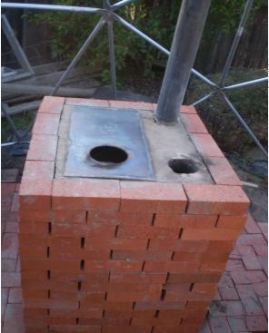
burn chamber. I have a circular plate of steel that covers the hole when the pot is not in place
